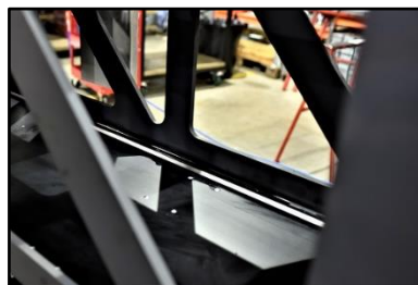
02.76 Bottom Rails for the wheels inside
