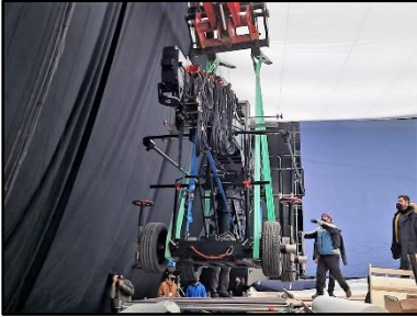
10.xx Lifting the crane.
